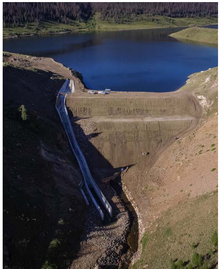
Continental Reservoir's spillway. Photo: Keith Holland
